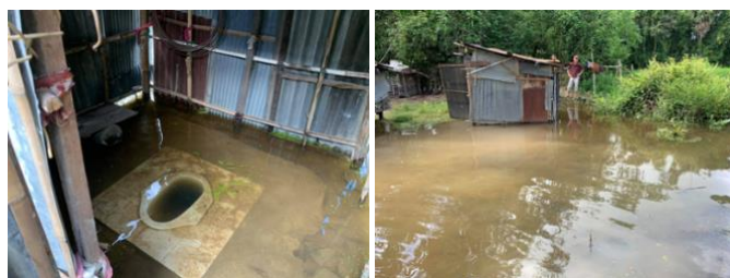
Figure 4: Flooding at one household that prevented its members from accessing or using their latrine
