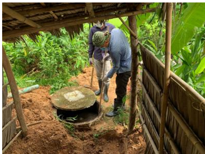
Figure 5: Measuring the sludge level within a pit
