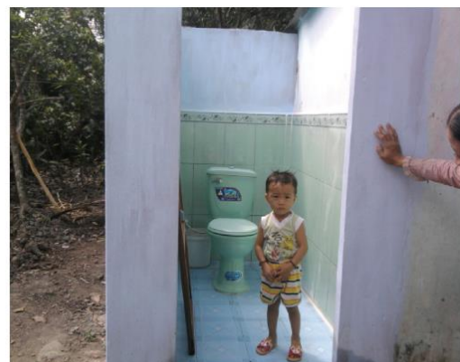
New toilet with septic system build with a CHOBA rebate
