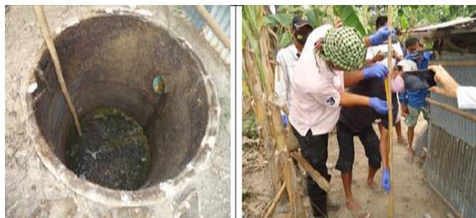
Figure 2: Measuring the sludge level within a pit
